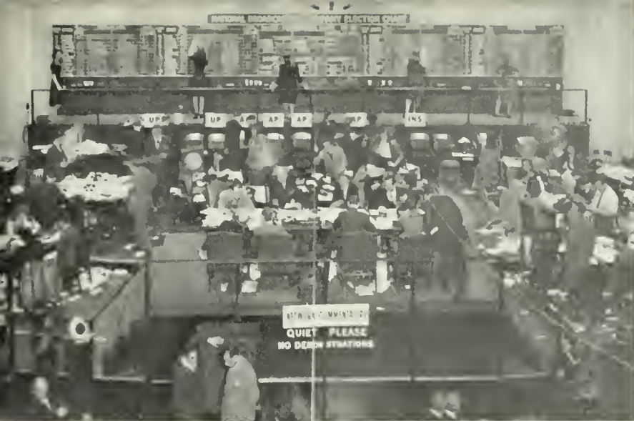
SCENE IN STUDIO 8H ON ELECTION NIGHT IN 1944. ACTIVITIES IN THE SAME STUDIO WILL BE INTENSIFIED THIS YEAR BY THE PRESENCE OF SEVERAL TELEVISION CAMERAS.
