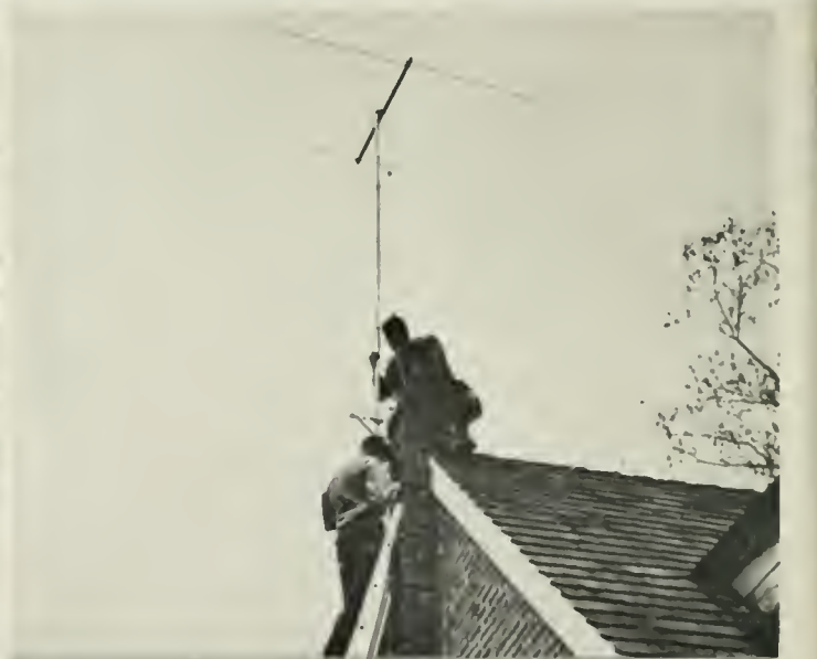
5. Using special rigging and supports, the antenna is clamped securely to the most suitable spot on the roof.
