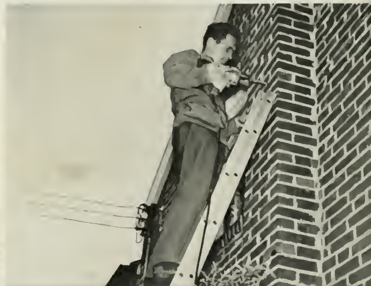
6. Holes are drilled in the side of the house to support hooks for the RCA "Bright-picture" tape which conveys signals to the receiver.
