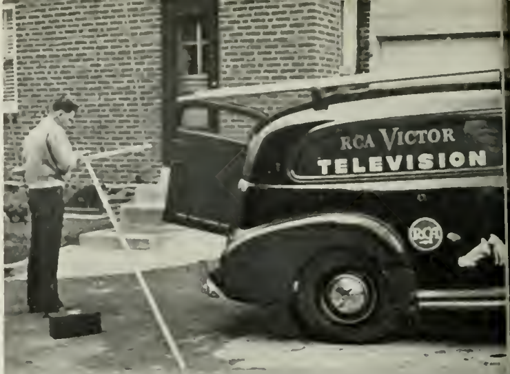
4. When the truck arrives at the customer's house, the RCA dipole receiving antenna is assembled on the ground before being erected on the roof.
