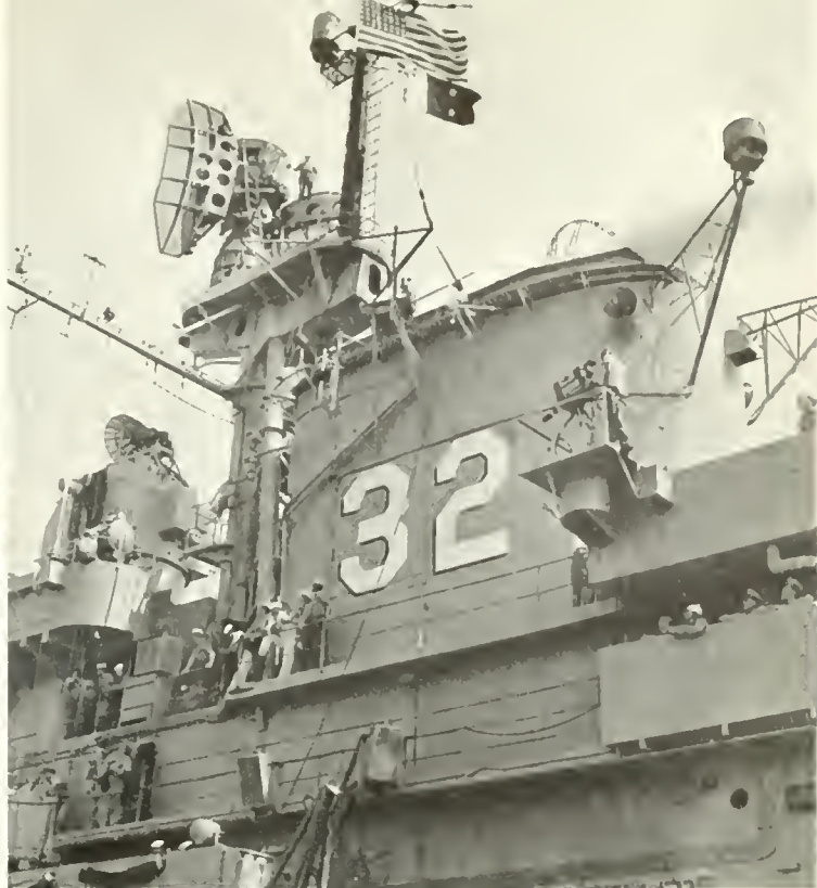
AGAINST A COLORFUL BACKGROUND OF ANTENNAS FOR RADAR AND OTHER SERVICES, A TELEVISION CAMERAMAN TRAINS HIS INSTRUMENT ON ACTIVITIES BELOW.
